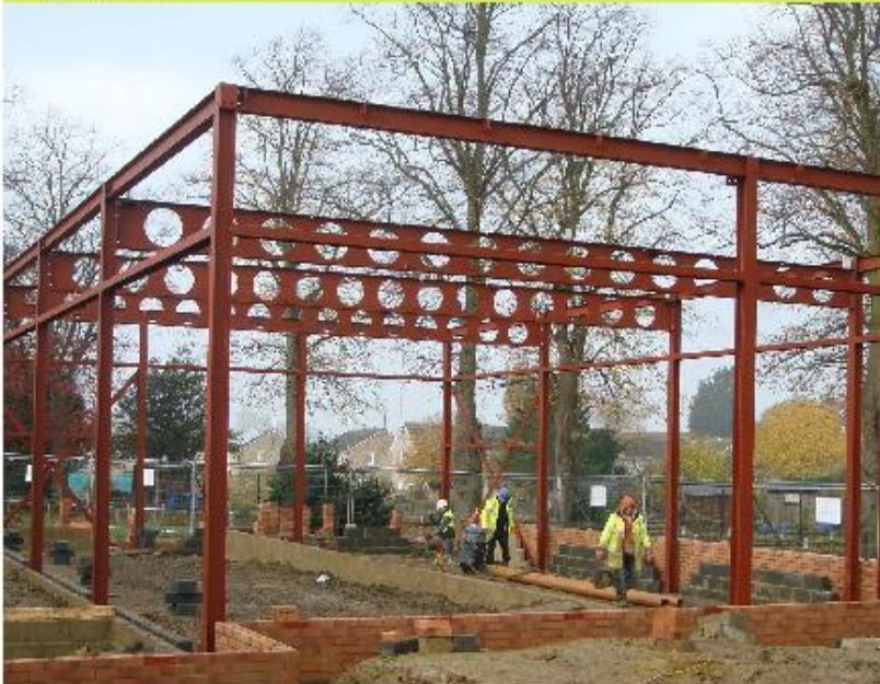
Benefits of CAT - Gym at Middleton Pool under construction
